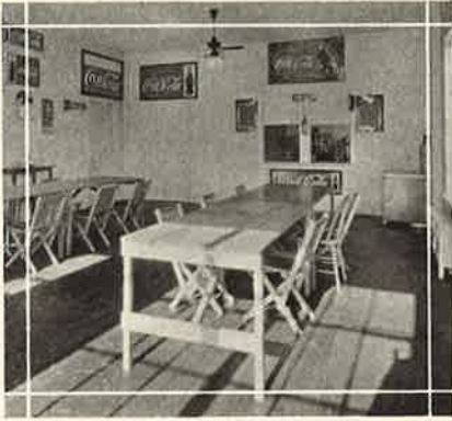
A portion of the assembly room, where advertising matter is also kept.
