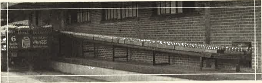
Truck unloading empties on roller conveyor which carries them into basement of building.
