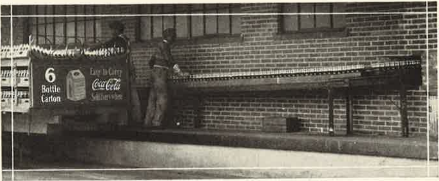
The same truck loading fulls from the roller conveyor just ahead of the one shown above.
