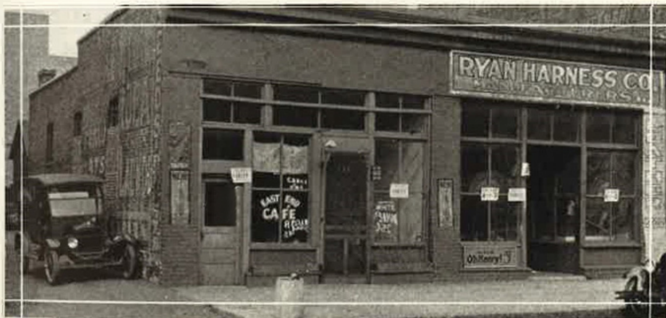
This is the site of the first home of the Birmingham Coca-Cola Bottling Co. It is located at 109 N. 24th St., in Birmingham, Ala. The building is now occupied by a cafe and a harness shop.
