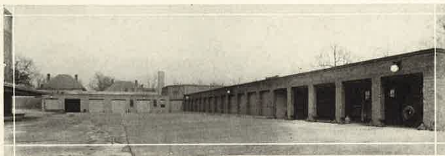
The truck and passenger car garage.
