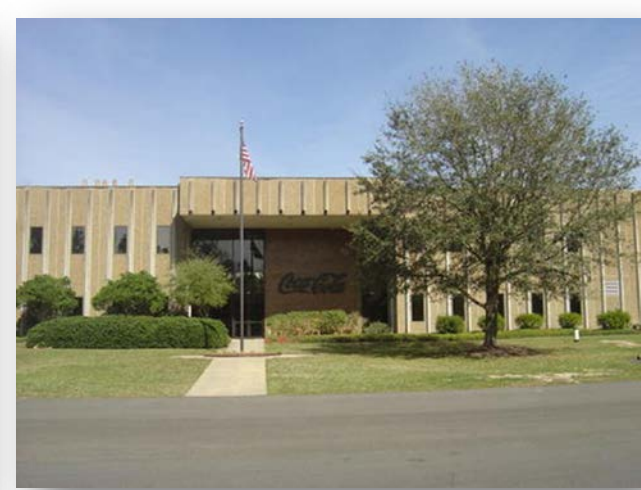
Hattiesburg Coca-Cola's Current Facility Located at 201 Coca-Cola Avenue, Hattiesburg, MS
