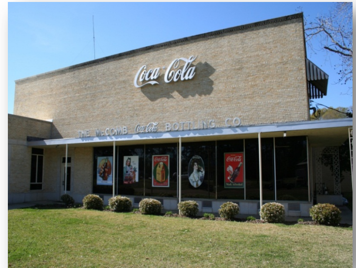
McComb Coca-Cola's Current Facility Located at 310 Presley Blvd. McComb, MS
