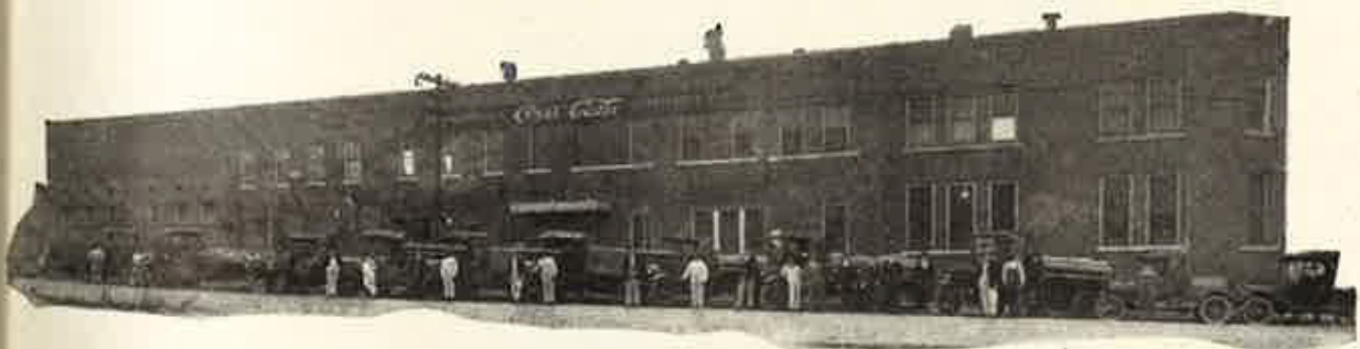
The third plant, constructed in 1908, was located at Avenue E and 22nd St., Birmingham. This plant served until the present masterpiece was built.
